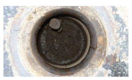
**OBSERVATION:** 3/4" IRON PIN (REBAR) IN MONUMENT BOX, NO TAG **MONUMENT REFERENCE:** 1/4 SECTION CORNER COMMON TO SECTIONS 28 & 29, T.1S., R.7E., M.D.B.&M.
