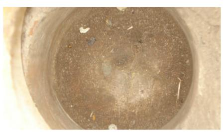
**OBSERVATION:** CHISELED CROSS IN CONCRETE (TOP OF IRRIGATION PIPE) IN MONUMENT BOX **MONUMENT REFERENCE:** SECTION CORNER COMMON TO SECTIONS 1 & 12, T.2S., R.7E. & SECTIONS 6 & 7,
