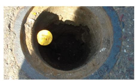
**OBSERVATION:** 3/4" IRON PIN (REBAR) WITH PLASTIC CAP STAMPED R.E. 14269 IN MONUMENT BOX
