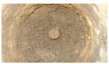
**OBSERVATION:** 5/8" IRON PIN (REBAR)IN MONUMENT BOX, NO TAG **MONUMENT REFERENCE:** SECTION CORNER COMMON TO SECTIONS 24 & 25, T.1S., R.7E. & SECTIONS 19 & 30,
