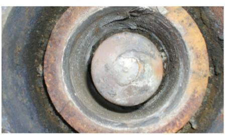
**OBSERVATION:** 2 1/4" BRASS DISK STAMPED S.J. CO LS 2239 ON IRON PIN IN MONUMENT BOX **MONUMENT REFERENCE:** 1/4 SECTION CORNER COMMON TO SECTION 25, T.1S., R.7E. & SECTION 30, T.1S.,
