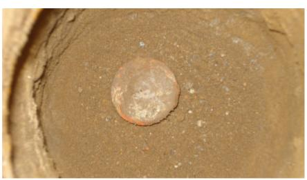
**OBSERVATION:** 2" BRASS DISK STAMPED S.J. CO. RE 1988, ON IRON PIN IN MONUMENT BOX **MONUMENT REFERENCE:** 1/4 SECTION CORNER COMMON TO SECTION 1, T.2S,. R.7E. & SECTION 6, T.2S.,
