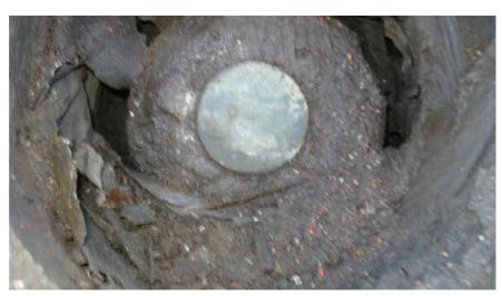
**OBSERVATION:** 2 1/2" BRASS DISK STAMPED LS 6314 ON CONCRETE CYLINDER IN MONUMENT BOX **MONUMENT REFERENCE:** SECTION CORNER COMMON TO SECTIONS 35 & 36, T.1S., & SECTIONS 1 & 2 T.2S.,
