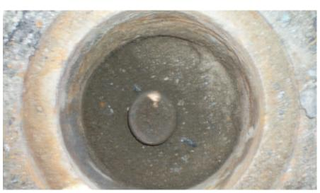
**OBSERVATION:** 2" IRON PIPE IN MONUMENT BOX, NO TAG, BOX 0.3' DOWN **MONUMENT REFERENCE:** 1/4 SECTION CORNER COMMON TO SECTIONS 27 & 28, T.1S., R.7E., M.D.B.&M.
