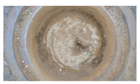
**OBSERVATION:** INDENTATION IN PAVEMENT, NO NAIL PER PREVIOUS SURVEY IN MONUMENT BOX **MONUMENT REFERENCE:** 1/4 SECTION CORNER COMMON TO SECTIONS 29 & 30, T.1S., R.7E., M.D.B.&M.
