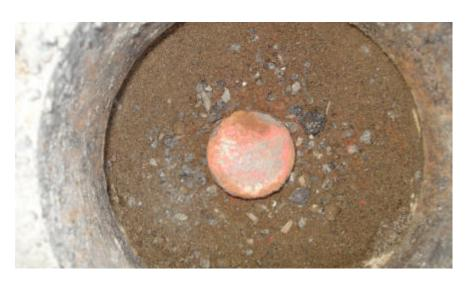
**OBSERVATION:** 2" BRASS DISK STAMPED LS 2239 ON IRON PIN IN MONUMENT BOX, BOX RIM 0.4' DOWN) **MONUMENT REFERENCE:** SECTION CORNER COMMON TO SECTIONS 25, 26, 35 & 36, T.1S,. R.7E., M.D.B.&M.
