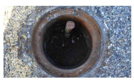
**OBSERVATION:** 3/4" IRON PIN (REBAR) IN MONUMENT BOX, NO TAG **MONUMENT REFERENCE:** 1/4 SECTION CORNER COMMON TO SECTIONS 21 & 28, T.2S., R.7E., M.D.B.&M.
