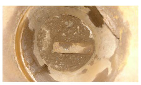
**OBSERVATION:** 1" IRON PIN, NO TAG, IN MONUMENT BOX, BENT HORIZONTALLY TO THE SOUTH **MONUMENT REFERENCE:** SECTION LINE COMMON TO SECTIONS 7 & 8, T.2S., R.7E., M.D.B.&M. AND CENTERLINE OF
