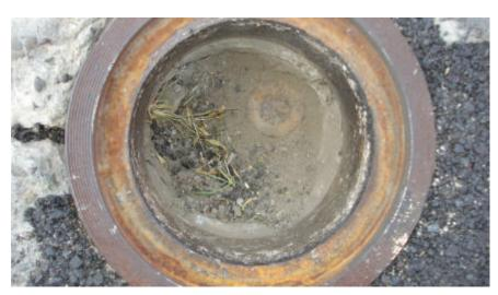
**OBSERVATION:** 2" WASHER & IRON PIN IN MONUMENT BOX , NO MARKINGS **MONUMENT REFERENCE:** 1/4 SECTION CORNER COMMON TO SECTIONS 11 & 12, T.2S., R.6E., M.D.B.&M. RECORDED REFERENCE: RS 33-133 (POINT NO. 208)(SJ CO. SURVEYORS MONUMENT IN MON. WELL)
