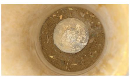
**OBSERVATION:** 2 1/4" BRASS DISK, STAMPED S.J. CO. RE 9338, ON IRON PIN IN MONUMENT BOX **MONUMENT REFERENCE:** SECTION CORNER COMMON TO SECTIONS 12 & 13, T.2S., R.6E. & SECTIONS 7 & 18,
