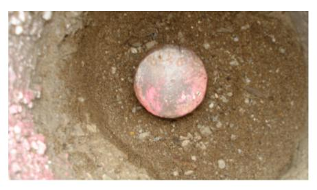
**OBSERVATION:** 2" BRASS DISK STAMPED S.J. CO. RE 9338 IN MONUMENT BOX. **MONUMENT REFERENCE:** SECTION CORNER COMMON TO SECTIONS 2, 3, 10 & 11, T.2S., R.7E., M.D.B.&M.
