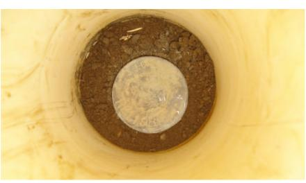
**OBSERVATION:** 2 1/4" BRASS DISK STAMPED S.J. CO., RE 11988 ON IRON PIN IN MONUMENT BOX **MONUMENT REFERENCE:** 1/4 SECTION CORNER COMMON TO SECTIONS 13, T.2S., R.6E. & SECTIONS 18, T.2S.,
