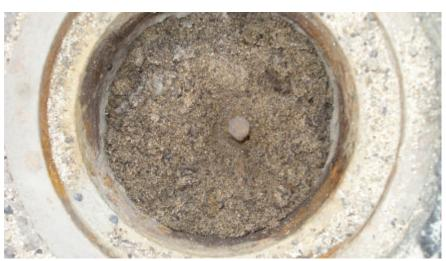
**OBSERVATION:** 1/2" IRON PIN (REBAR) IN MONUMENT BOX, NO TAG **MONUMENT REFERENCE:** SECTION CORNER COMMON TO SECTIONS 15, 16, 21& 22, T.2S., R.7E., M.D.B.&M.
