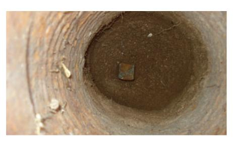
**OBSERVATION:** 1" SQUARE ROD IN MONUMENT BOX, NO TAG **MONUMENT REFERENCE:** SECTION CORNER COMMON TO SECTIONS 8, 9, 16 & 17, T.2S., R.7E., M.D.B.&M.
