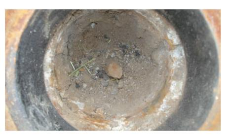
**OBSERVATION:** 3/4" IRON PIN (REBAR) IN MONUMENT BOX, NO TAG **MONUMENT REFERENCE:** SECTION CORNER COMMON TO SECTIONS 21, 22, 27 & 28, T.2S., R.7E., M.D.B.&M.
