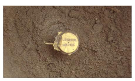
**OBSERVATION:** 3/4" IRON PIPE WITH PLASTIC PLUG STAMPED TURNROSE LS 7454, 1.5' DOWN
