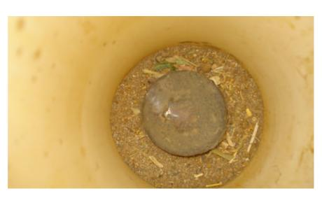
**OBSERVATION:** 2 1/4" BRASS DISK STAMPED S.J. CO., RE 11988, ON IRON PIN IN MONUMENT BOX **MONUMENT REFERENCE:** SECTION CORNER COMMON TO SECTIONS 13 & 24, T.2S., R.6E. & SECTIONS 18 & 19,
