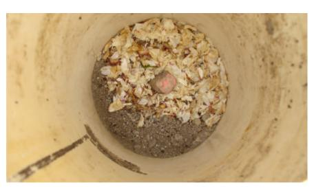
**OBSERVATION:** 3/4" IRON PIN (REBAR) IN MONUMENT BOX, 1.2' DOWN, NO TAG **MONUMENT REFERENCE:** 1/4 SECTION CORNER COMMON TO SECTIONS 14 & 23, T.2S., R.7E., M.D.B.&M.
