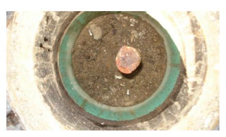
**OBSERVATION:** 1" IRON PIN (REBAR) IN MONUMENT BOX, NO TAG **MONUMENT REFERENCE:** 1/4 SECTION CORNER COMMON TO SECTIONS 7 & 8, T.2S., R.7E., M.D.B.&M.
