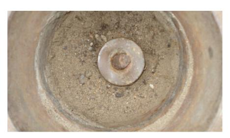
**OBSERVATION:** 2 1/2" WASHER STAMPED S.J. CO. LS 2239 ON IRON PIN IN MONUMENT BOX **MONUMENT REFERENCE:** SECTION CORNER COMMON TO SECTIONS 14, 15, 22 & 23, T.2S., R.7E., M.D.B.&M.
